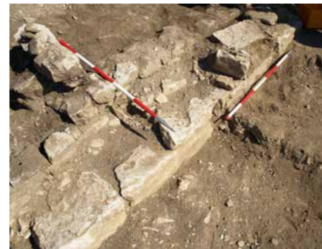
Sl. 15. Proširenje temeljne stope zida 10d | Fig. 15. Extension of the base level of the wall 10d
