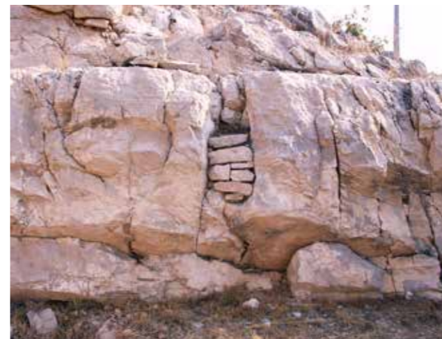
Sl. 21. Popuna zida prostorije P 12 | Fig. 21. Filling of the wall in Room P 12
